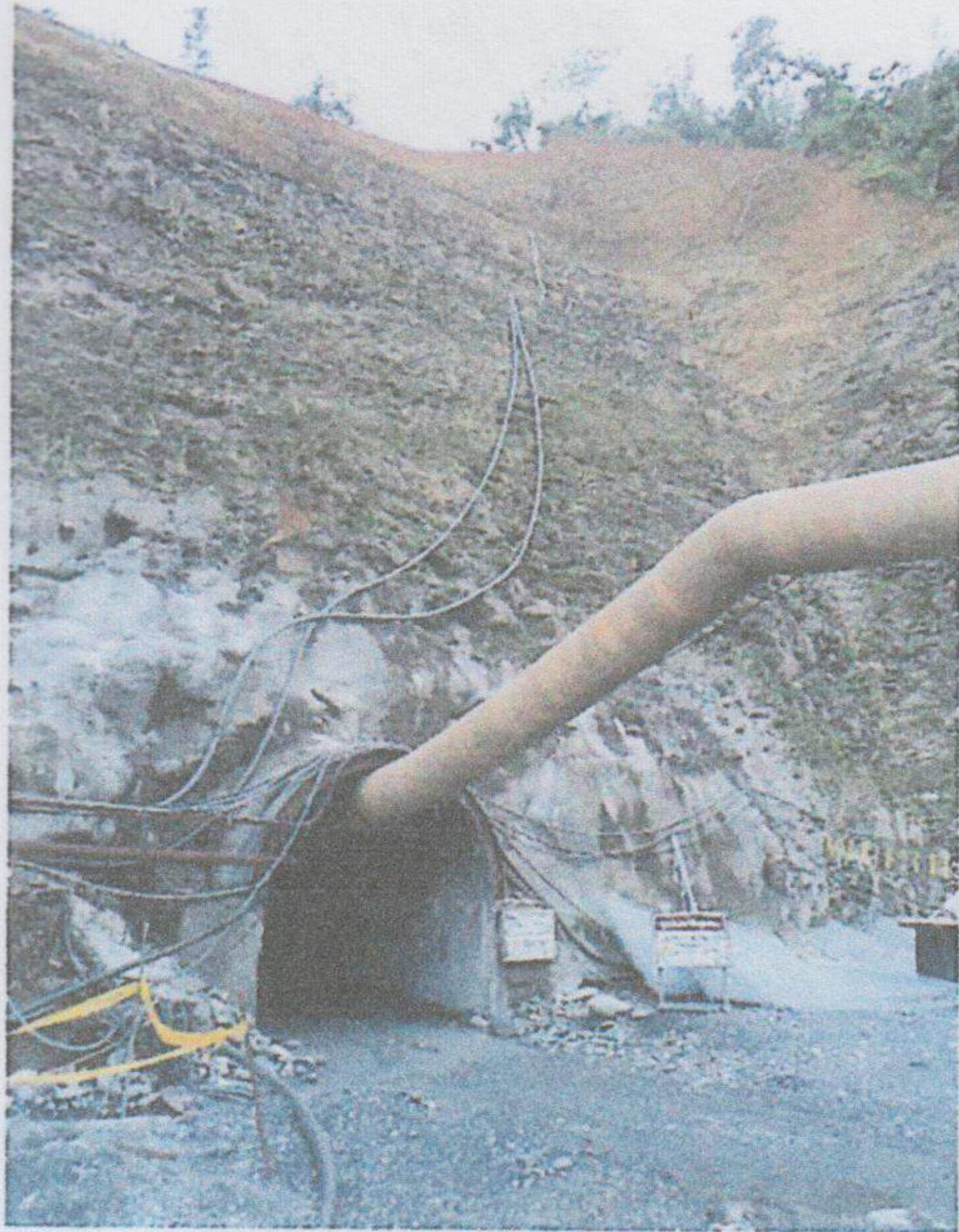
Photo 1 -Outlet Portal of the main tunnel
