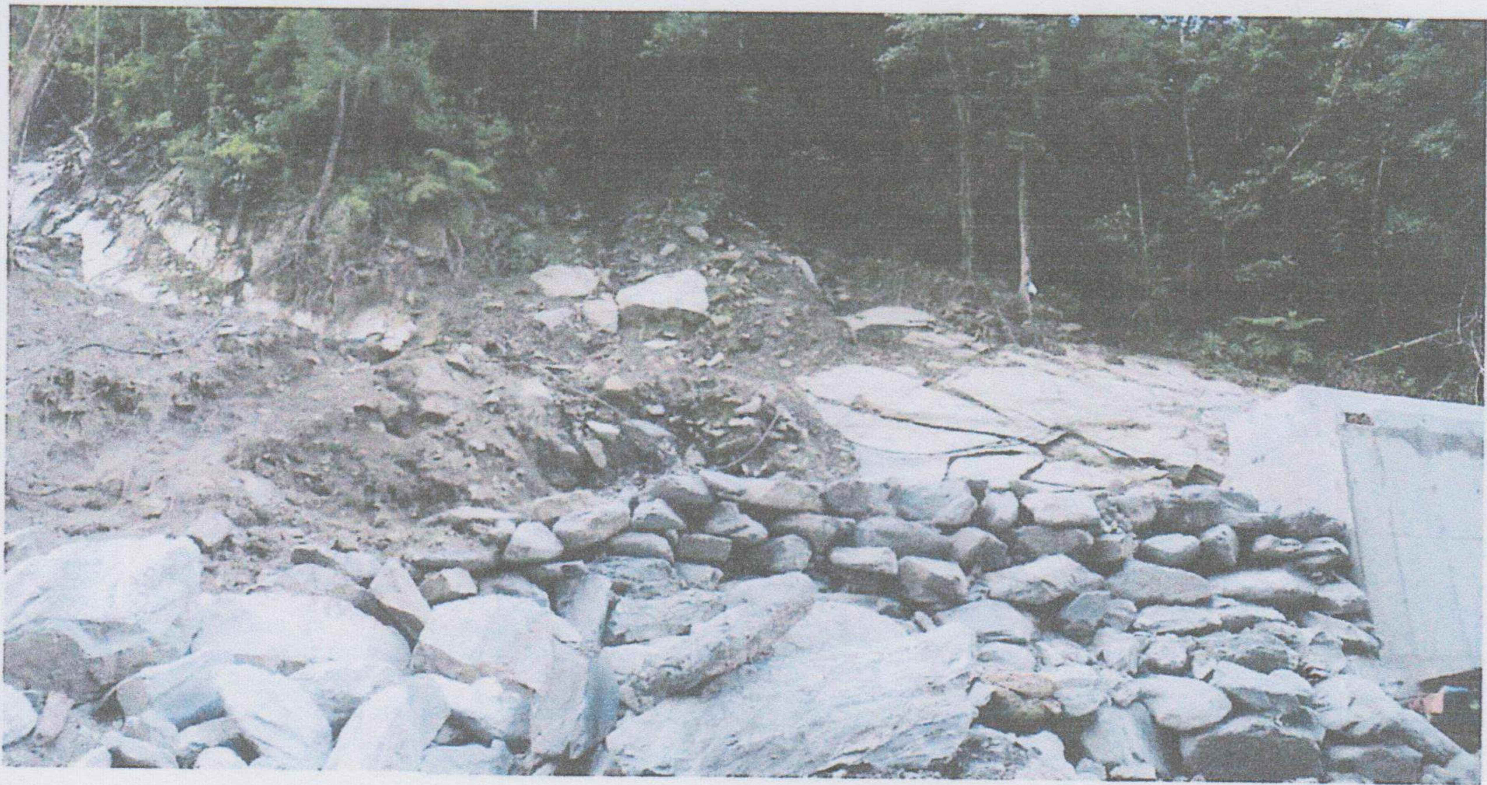
Photo 6- Deposit of rocks, soil, and debris overlying bedrock that prone to debris slide during incessant rains.
