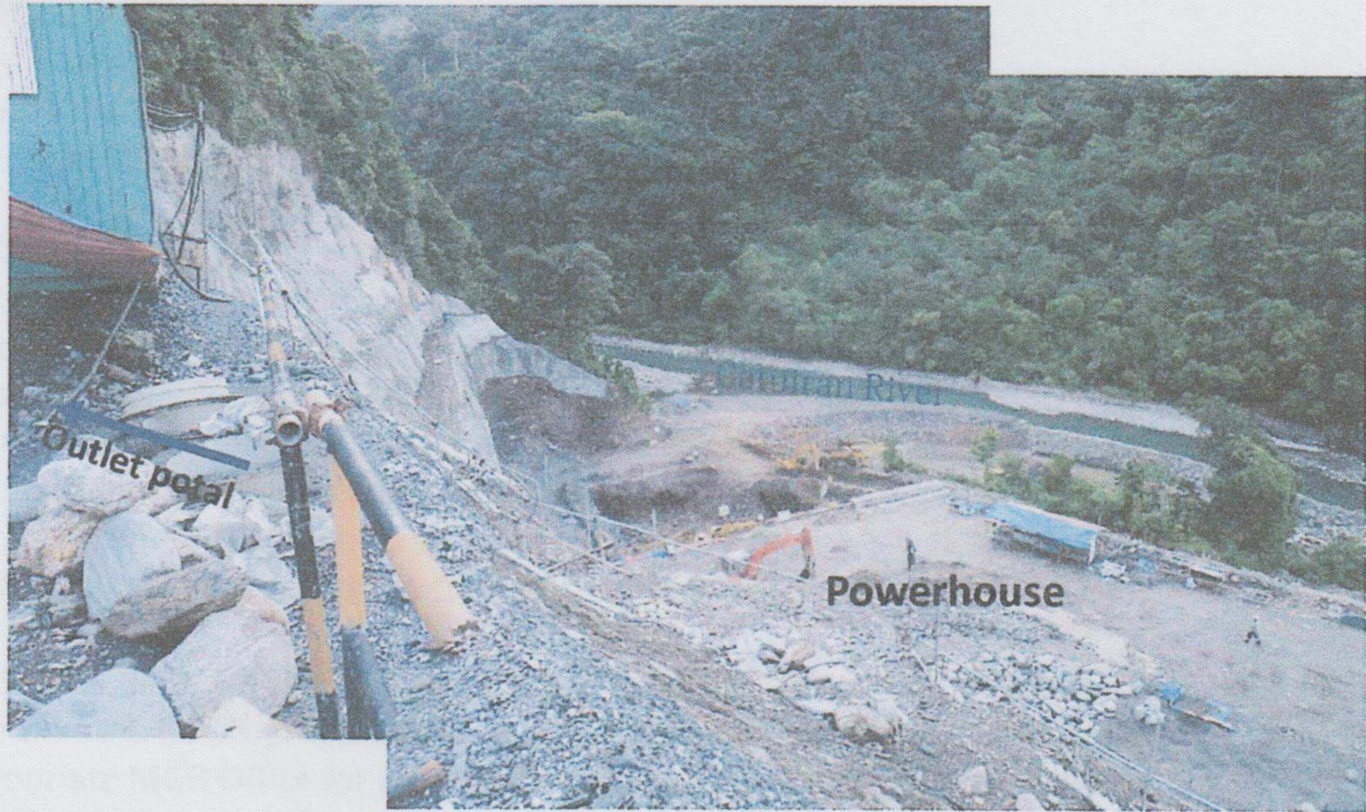
Photo 7 - Massive stabilization is underway at the Powerhouse area
