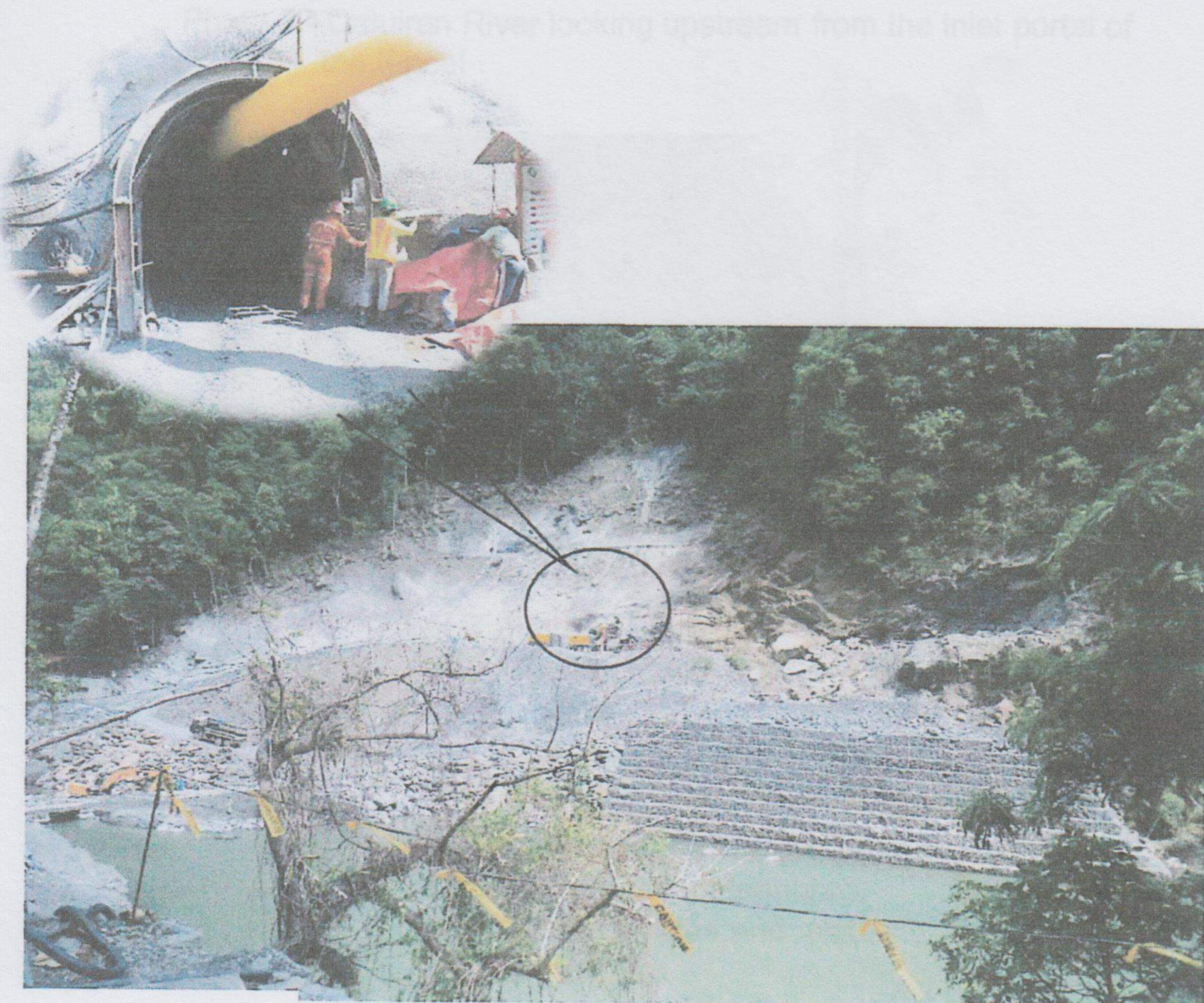
Photo 2 - Inlet Portal of the tunnel
