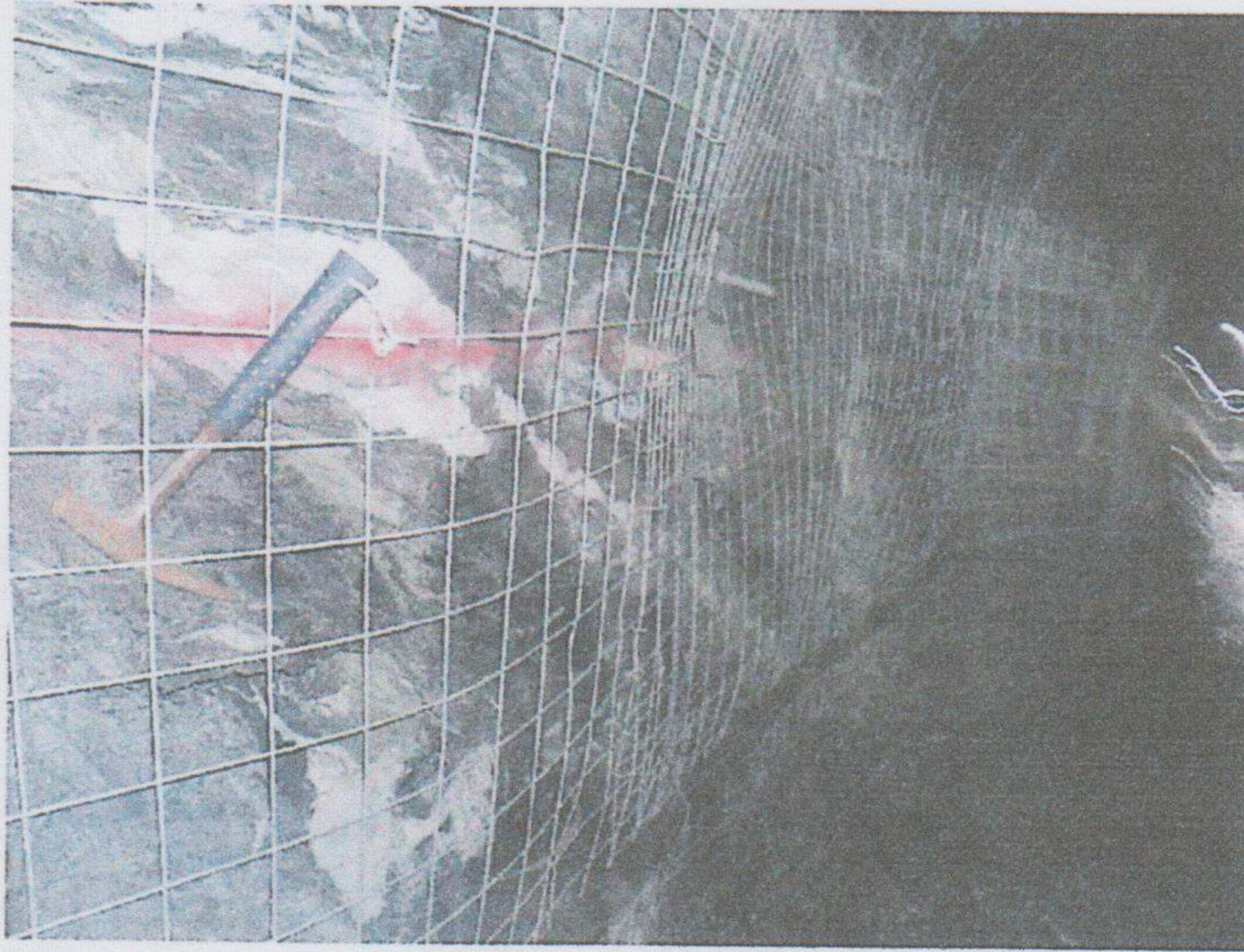
Photo 5 – Quartz lenses observed inside the tunnel near the inlet portal.
